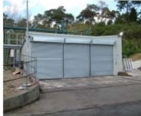
Grit Skip Enclosure (East)
