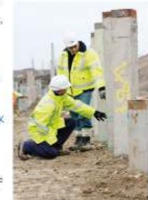
Assistant Engineer James Clark (left) inspects the piling with a representative from Black & Veatch.
