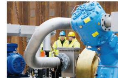
The new methane gas compressor will help generate renewable energy. Photographs on pages 1 and 2 courtesy of Nick Keane.
